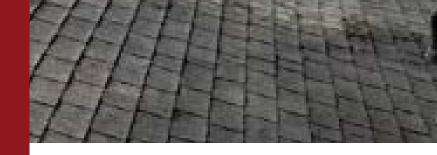
The sun's ultraviolet radiation threatens a roofing system's long-term health and functionality. Oxidation also begins to occur from day 0, further weakening the fibers in shingles and leading to their gradual breakdown.
